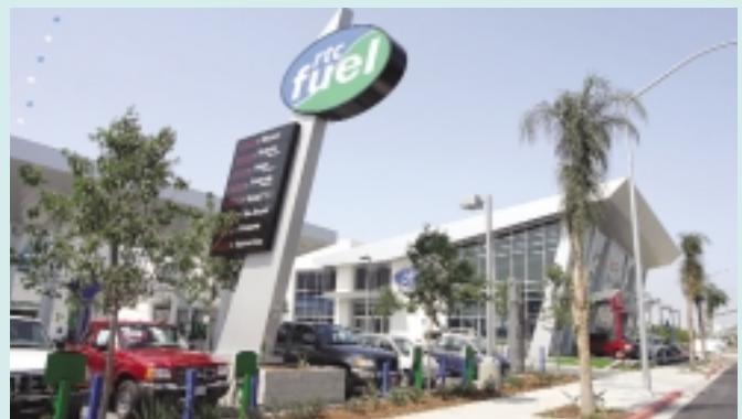
Regional Transportation Center
